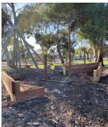
The new 'Shipwrecked' boat is almost finished
